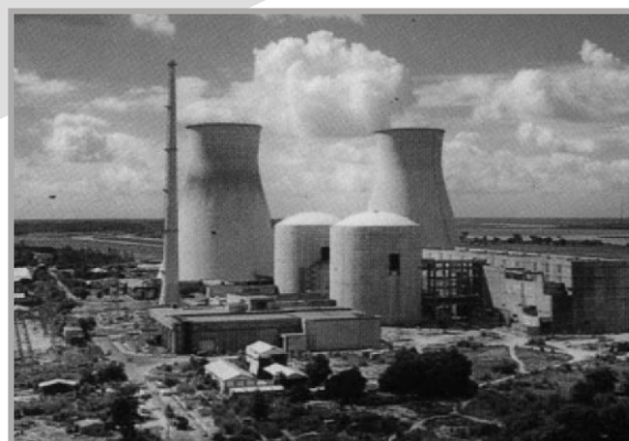
Narora Atomic Power Station
