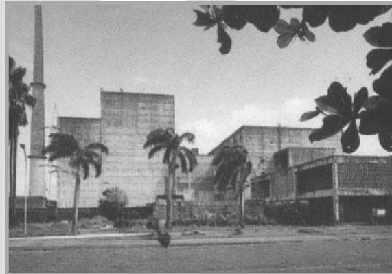
Tarapur Atomic Power Station
