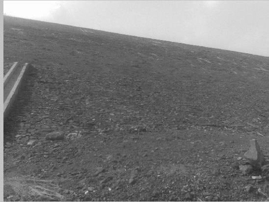
Stone lining on the tailings dam exterior for structural integrity
