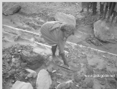
An old man showing the tailings pipe leak
