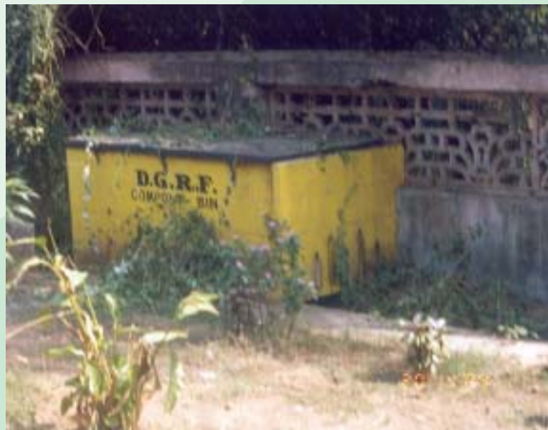
The segregated waste is composted in specially constructed bins that are placed at street corners or even above storm drains, as shown here.
