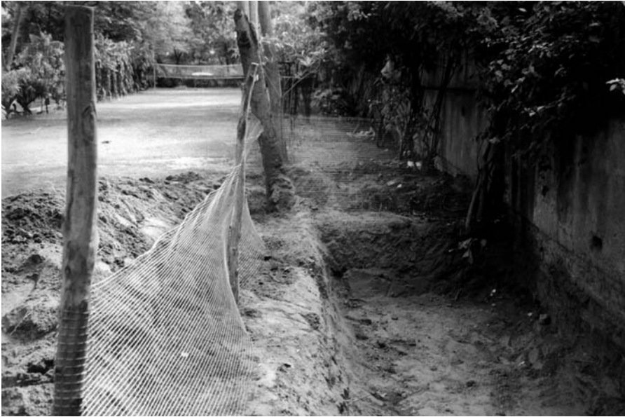
Natural pits were dug for aerobic composting of the waste.
