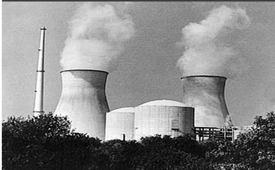
AN ATOMIC POWER STATION
