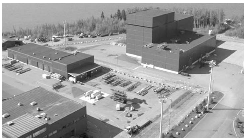
Spent fuel storage
